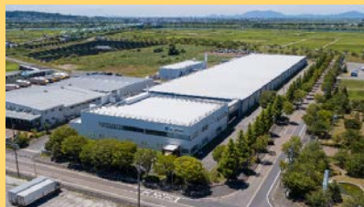
Kyogase Plant (Agano City, Niigata Pref.)
