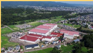
Arai Plant (Myoko City, Niigata Pref.)
