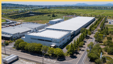
Kyogase Plant (Agano City, Niigata Pref.)
