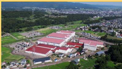
Arai Plant (Myoko City, Niigata Pref.)
