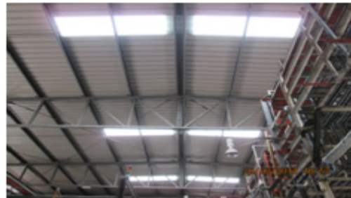
Transparent plates in the ceiling
