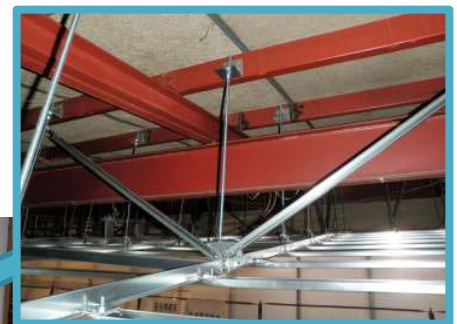
Aseismic frame in the ceiling
