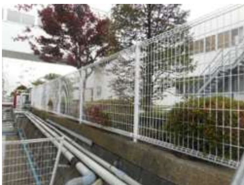
Installing fences to prevent falls
