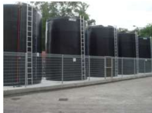
Large-scale water storage tank
