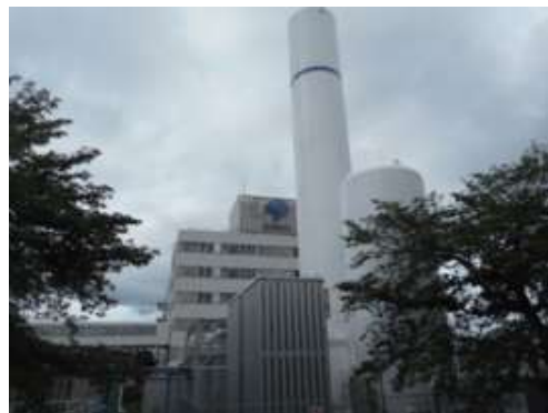
Nitrogen supply facilities
