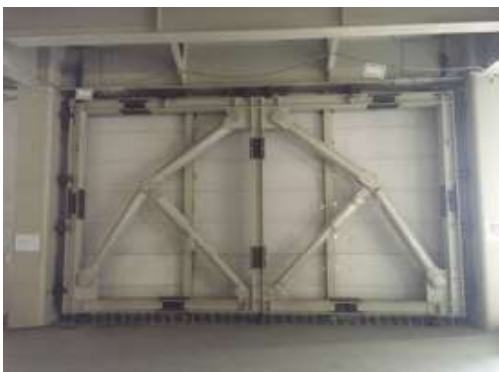
Toggle-brace-damper quake control devices
