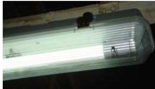
LED lamp with cover installed
