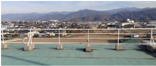
Rooftop with a fence installed
