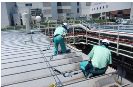
Working on a roof while attached to the Safe Slider
