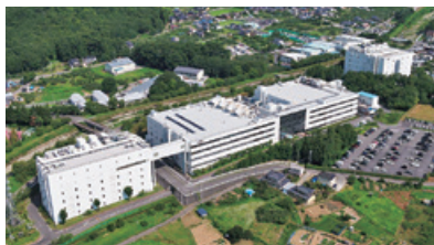
Wakaho Plant in Nagano City, Nagano Prefecture
