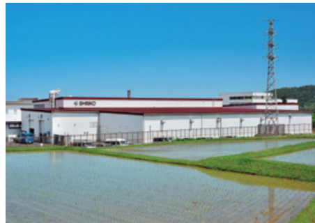
New facilities at the Arai Plant
